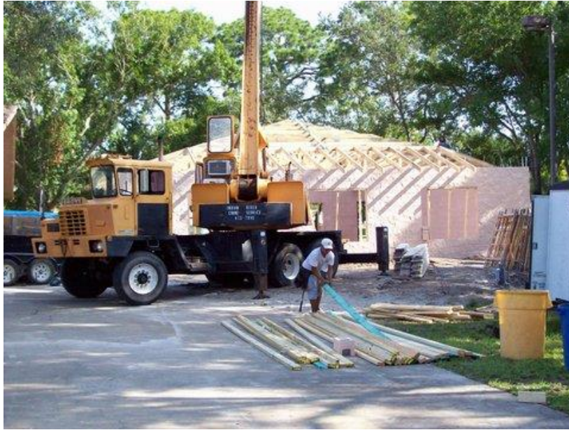
Preschool under construction summer 2007.
