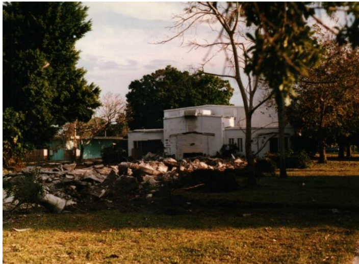
Downtown church building demolition on site of Main County Library.
